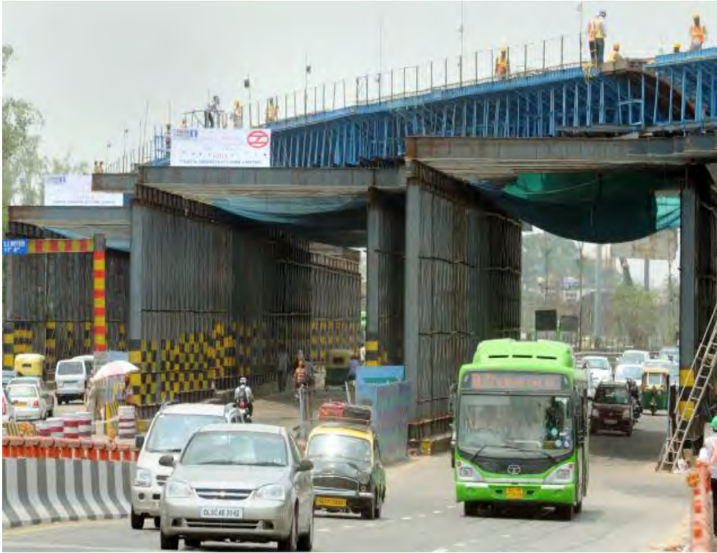
Construction underway in 2009 for the high speed railway line connecting New Delhi railway station with the international airport.
