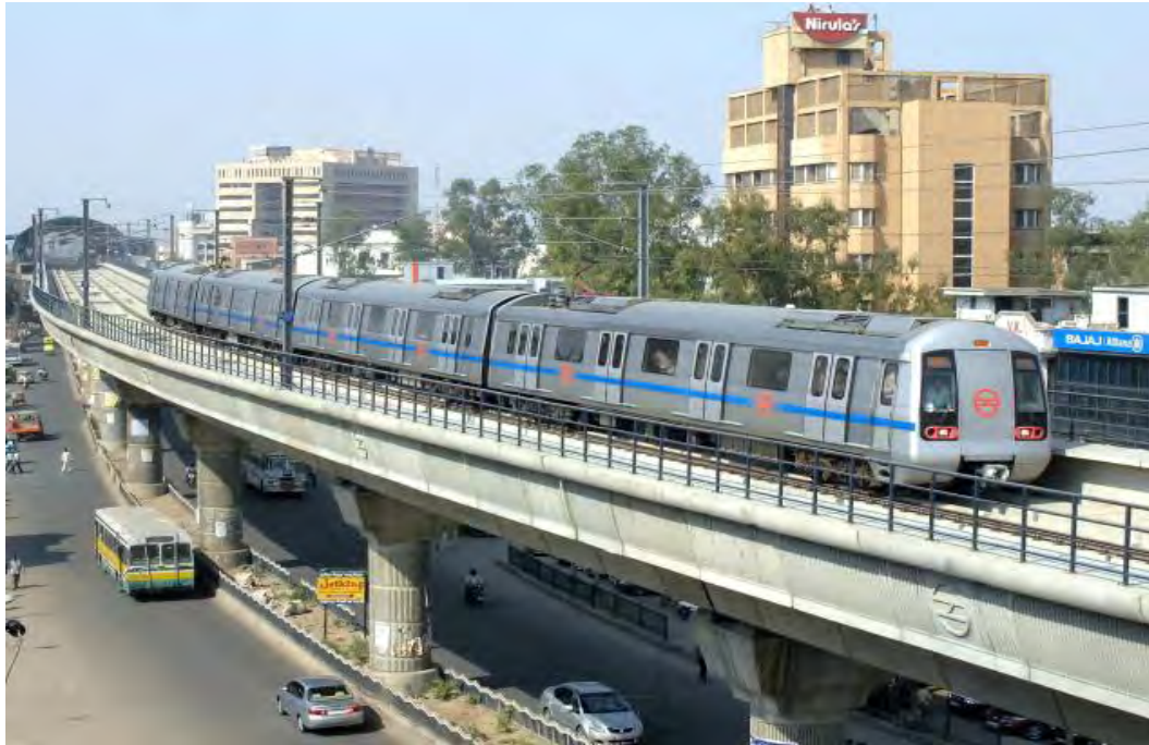
The Anand-Vihar line, the fourth on the Delhi Metro network, opened January 2010
