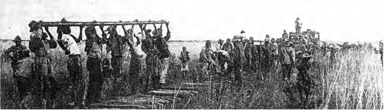
Construction of the Otavi Railway.
