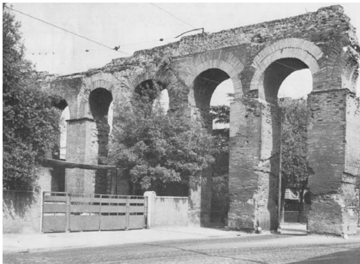
Photograph C Part of the Aqua Julia on the Esquiline Hill in Rome (Source: Open University Press/Fototeca Unione)
